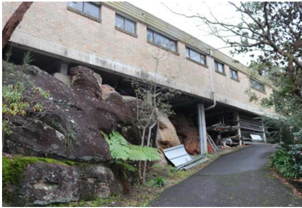
Figure 31: South-western c.1980s building, supported on concrete piers above sandstone outcrop
